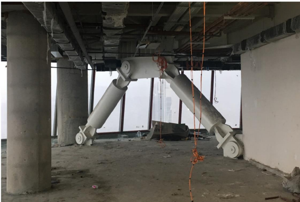
Figure 3.3 BRB-outrigger system
